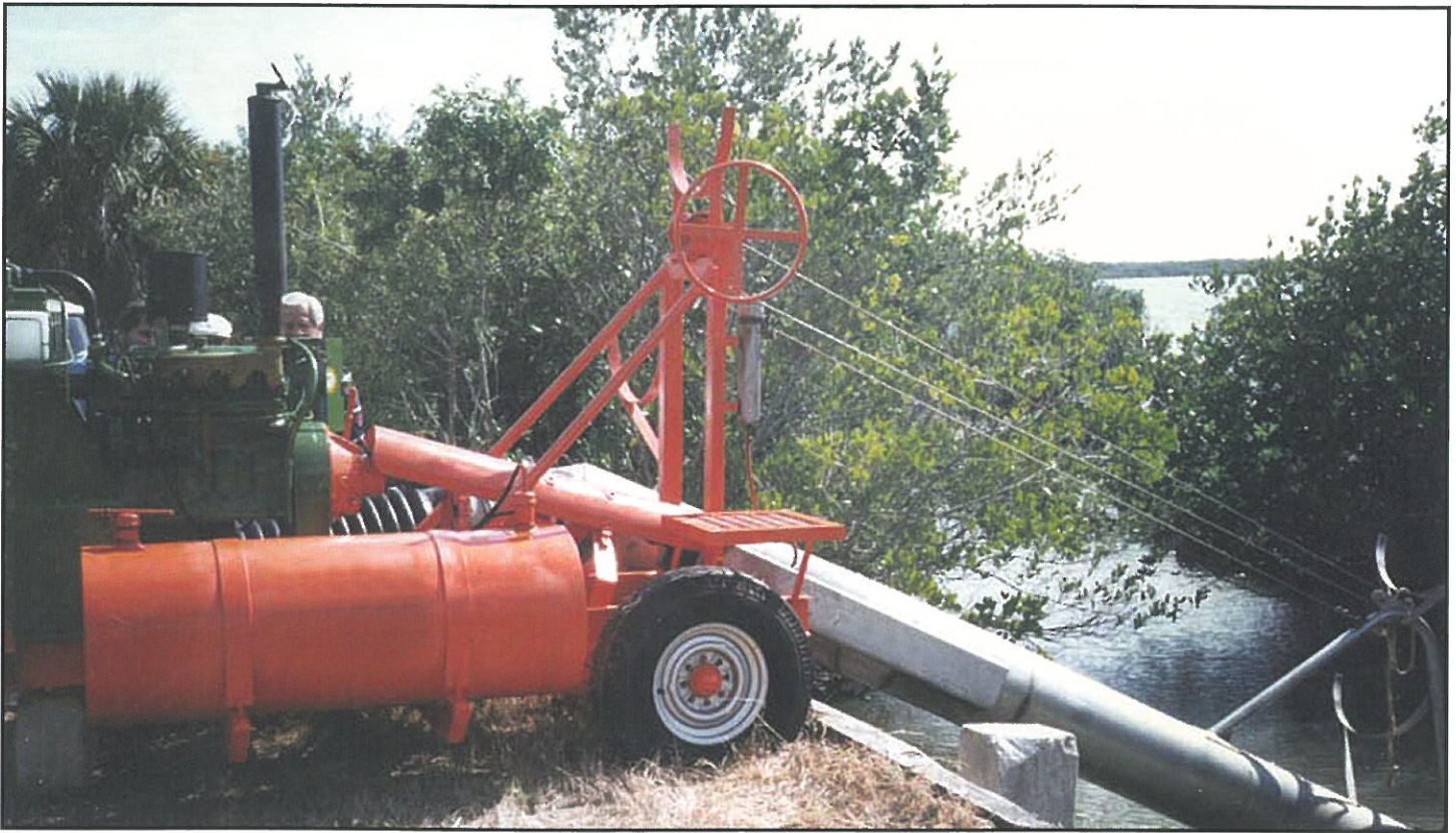
FIELD ACCEPTANCE TESTING OF STAINLESS STEEL AXIAL FLOW PUMP FOR SALT WATER APPLICATION
